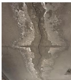
Fig. 1. Crack on soffit of slab
