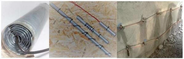
ZLRA is capable, of stopping and preventing corrosion of reinforcement within chloride contaminated or carbonated structures, preventing the need for removal and replacement of sound, undamaged chloride contaminated or carbonated concrete.
