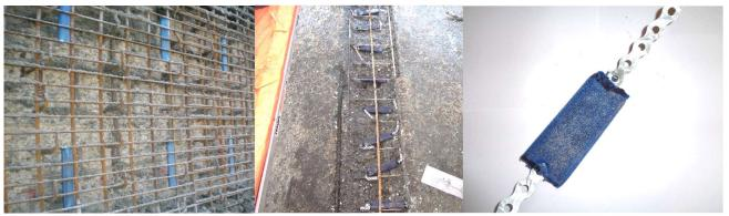
Where installed with monitoring facilities, ZLDA can be monitored and evaluated against the cathodic protection criteria listed within BS EN ISO 12696.
