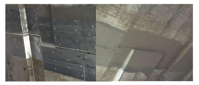
When installed onto the surface of atmospherically exposed concrete and electrically connected to the embedded reinforcement, ZLA provides active corrosion protection (**cathodic protection**) to the embedded reinforcement without the need for external AC or DC power.
