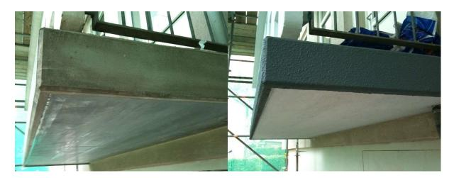
It is suitable for use on **high risk elements** like pre-stressed and post tensioned structures, as it will not exceed the potential limits listed within BS EN ISO 12696, and requires no further potential limitation or control during operation.
