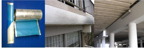
When connected to the embedded reinforcement and in contact with the concrete surface, the zinc foil corrodes at the humectant/activator/adhesive layer and provides **galvanic cathodic protection** to the embedded reinforcement.
